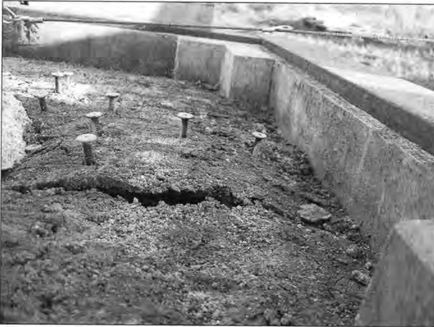
Figure 167 – Soil Bulging Behind Pile (115-mm Pile in Glacial Till)
