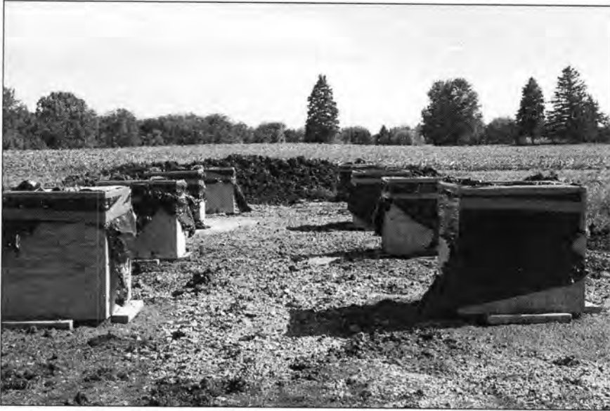
Figure 49 – Prepared Soil Forms
